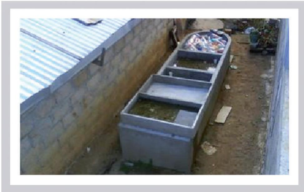
**Tank with laminated siphon (TLS).** The TLS is a hydraulic structure (tank) used to supply water intermittently to agricultural parcels (up to one hectare) small home gardens. This system has a discharge tube in the shape of a laminated siphon, which can save large amounts of water (up to 50 out of every 100 liters used) compared to continuous surface irrigation. The fundamental equation governing its intermittency for a constant flow input is:
